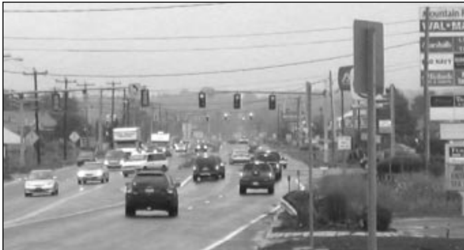
A 4-lane intersection, approximately 1/2 mile west of this 5-lane intersection at Mountain Farms Mall, is planned in front of the new Lowe's on Route 9 in Hadley. Between these two intersections, Route 9 will still narrow to 2 lanes.
